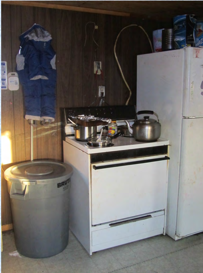
Cooking stove with no range exhaust
